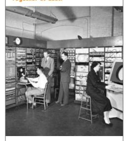
MIT's Whirlwind, which had been completed five years earlier, becomes the first computer in the world to allow its users to enter commands through a keyboard. Previously, all input was accomplished through dials, switches, and/or punch cards.
